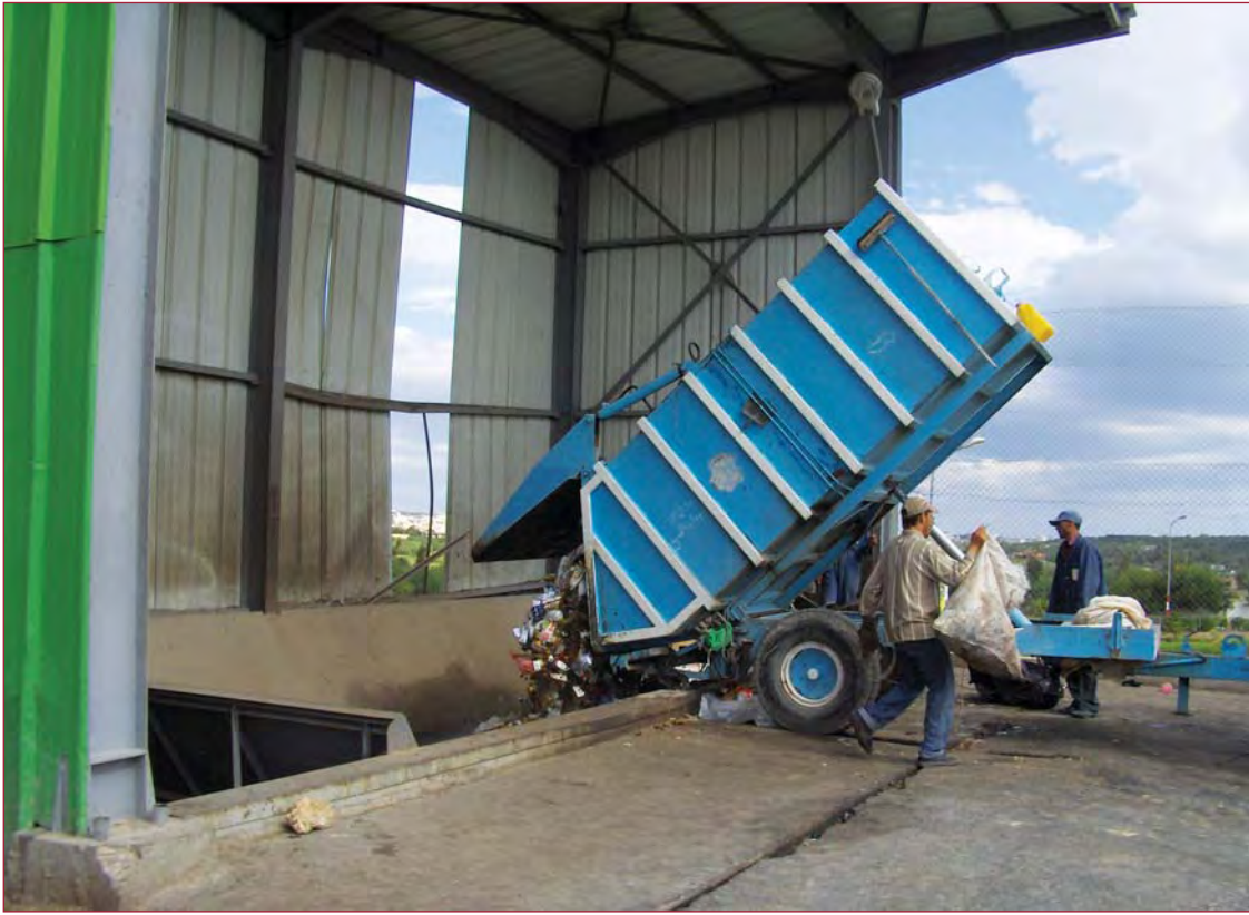
Transfer station in Sousse, Tunisia
