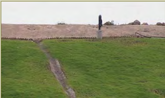
Gas venting pipe on waste dump
