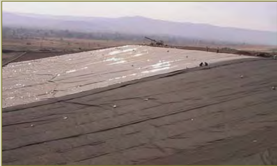
Laying HDPE liner
